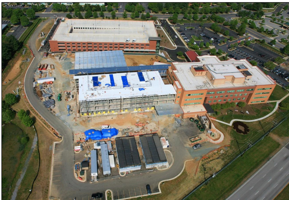
Figure 7 - An arial progress photo taken on April 21, 2012 shows the temporary roof just 12 days after its construction began. Take notice that there is no framing on the east façade. Image courtesy of DPR Construction.
