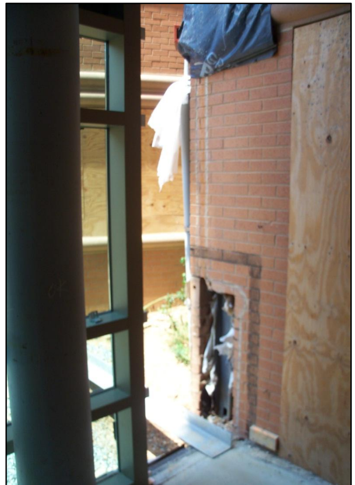
Figure 6 - Photograph taken from the interior of the addition looking at the corner of the existing building. The challenge is going to be demolishing small areas of existing facade and tying Air/Vapor Barrier to AVB behind that facade which will be getting opened. Personal photograph taken by Chris Pozza.
