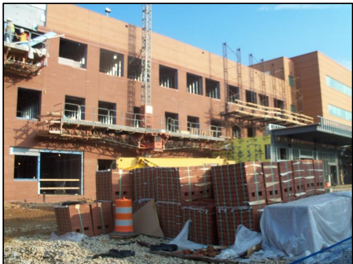
Figure 3 - The east elevation is shown almost completed. A Fraco lift can be seen in the center, with a Mason King manual cranked scaffold equipment sits on the canopy roof. Notice the amount of space currently taken up by the mason subcontractor. Personal photograph taken by Chris Pozza.
