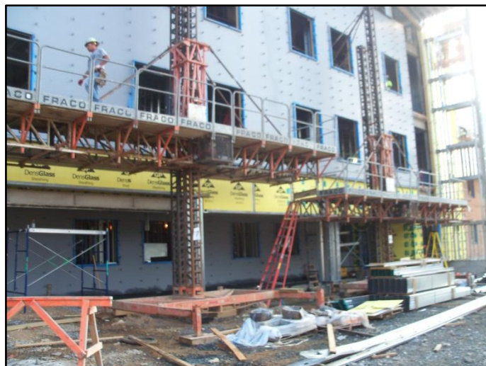
Figure 4 - Image taken the same day as Figure 10. Masons preparing for the next phase at the south elevation. Work can never take place underneath Fraco Lifts. Personal photograph taken by Chris Pozza.
